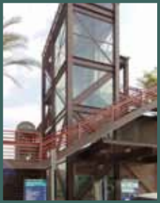
Light Rail Stations
